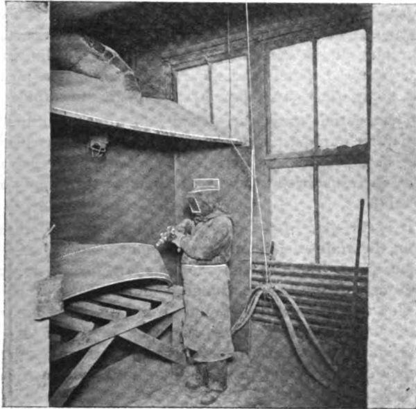
The old style sand-blast. The operator is free to discard his headgear when he finds it cumbersome
